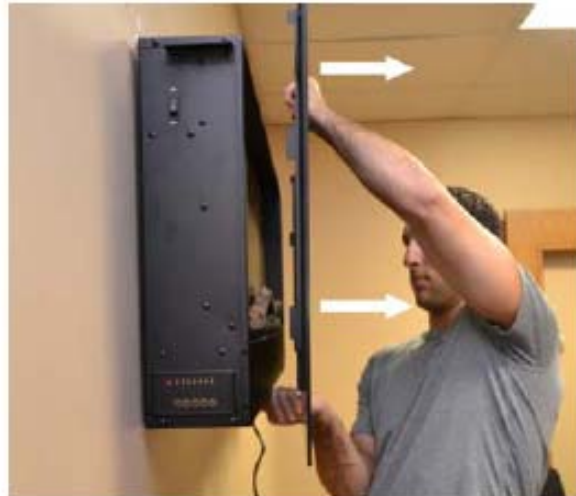
b. pull glass panel away from wall
